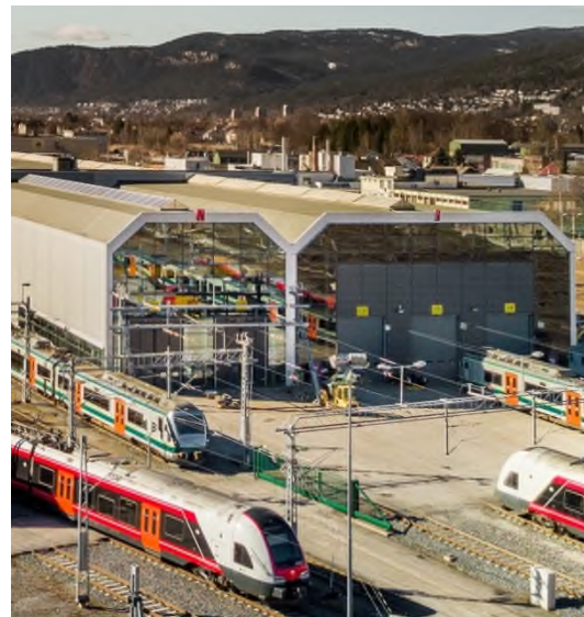
Bane NOR Eiendom's Maintenance hall in Drammen, Norway
