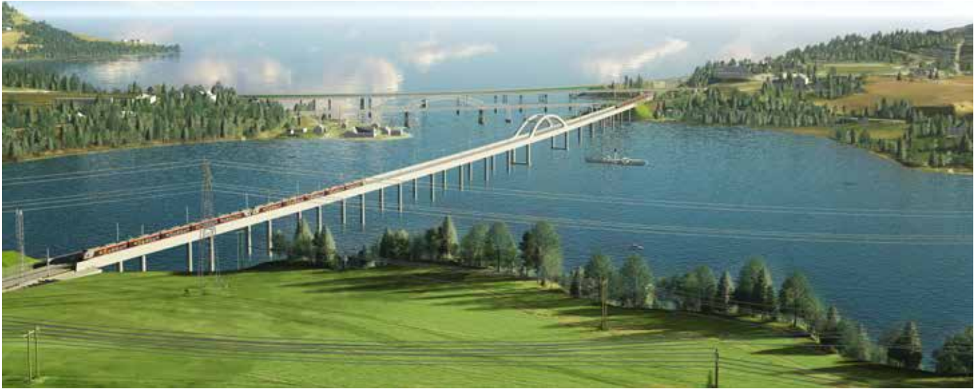
At 836 metres long, the Minnevika Bridge will be the longest railway bridge in Norway, until the completion of Tangenvika Bridge
