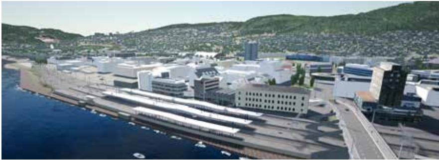
The railway station in Drammen city will be rebuilt with new platforms and tracks
