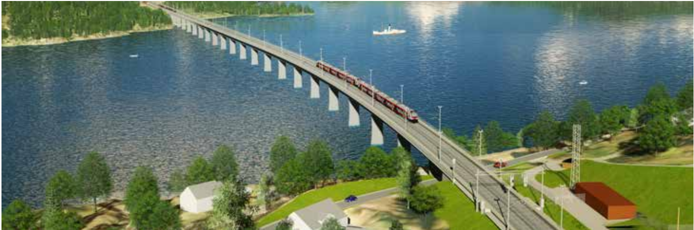
Tangenvika Bridge (1070 m) will be the longest railway bridge in Norway when it's completed
