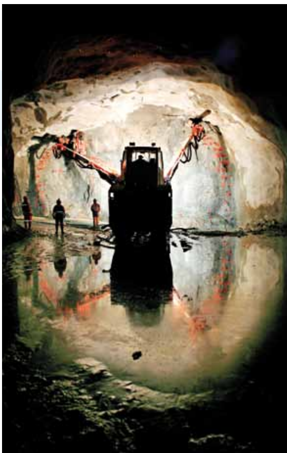
Tunneldriving. Foto: Hilde Lillejord/ Jernbaneverket
